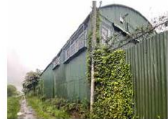
A5 Shed / Storage Building
