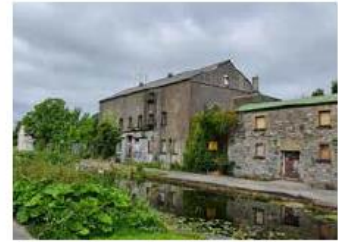
A3 Concrete Mill Building
