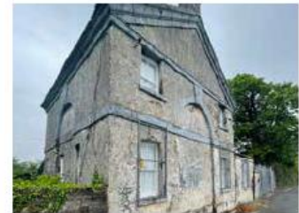
A4 Lock Keeper House
